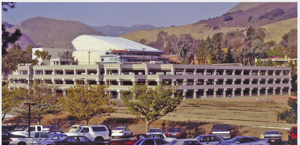
Parking structure at Cal Poly San Luis Obispo to serve daily campus commuters.
